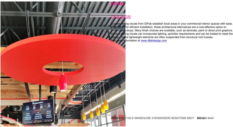
truction-drops. Many finish choices are available, such as laminate, paint or direct print graphics. lling clouds can incorporate lighting, sprinkler requirements and can be treated to meet fireese lightweight elements are often suspended from structural roof trusses. information at <a href="https://www.dfabdesign.com">www.dfabdesign.com</a>
